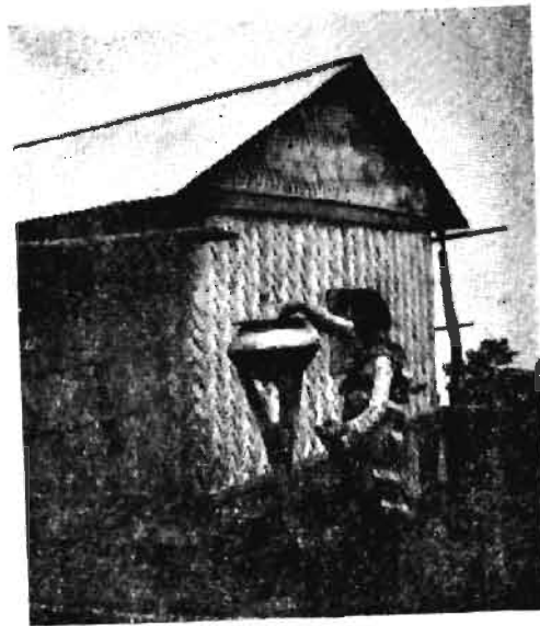
Reservoir of rain water. Observe the bamboo pipe propped below the eaves
